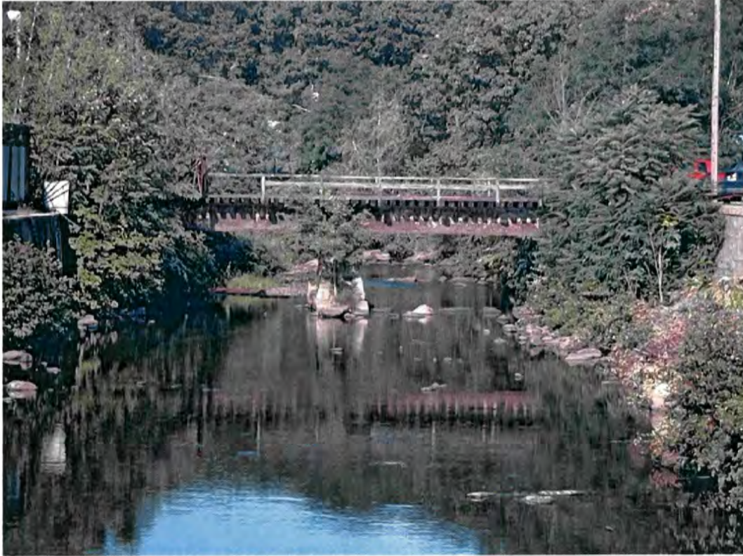
Photo 14: View upstream from Daniels Street (railroad bridge in center).
