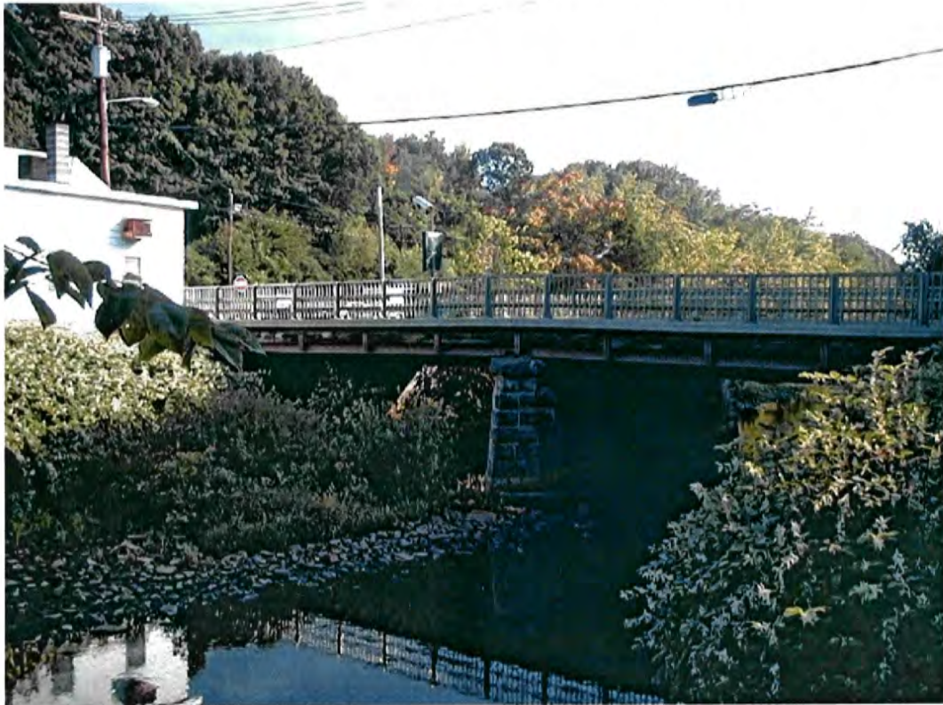
Photo 15: View of upstream side of Oak Hill Road bridge.
