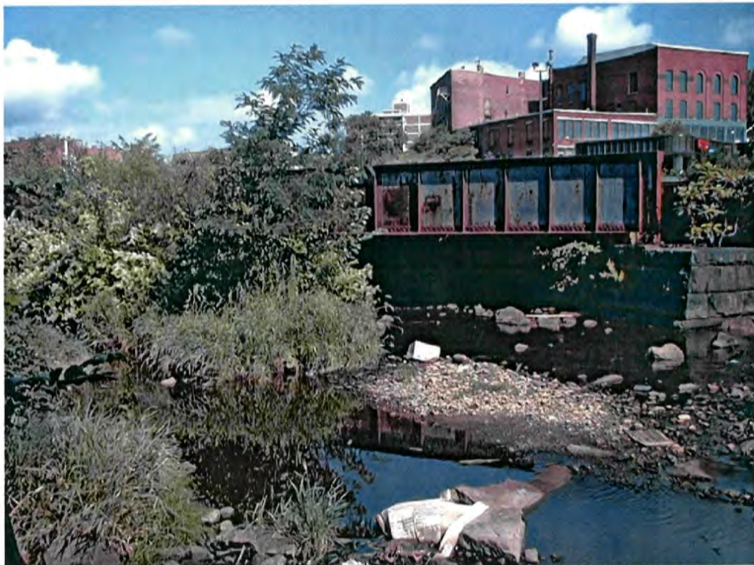
Photo 6: View upstream from below Laurel Street (railroad bridge in center).
