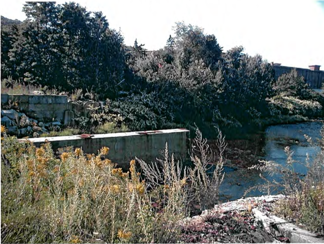
Photo 13: View upstream from Sheldon Street (pier supported demolished building).
