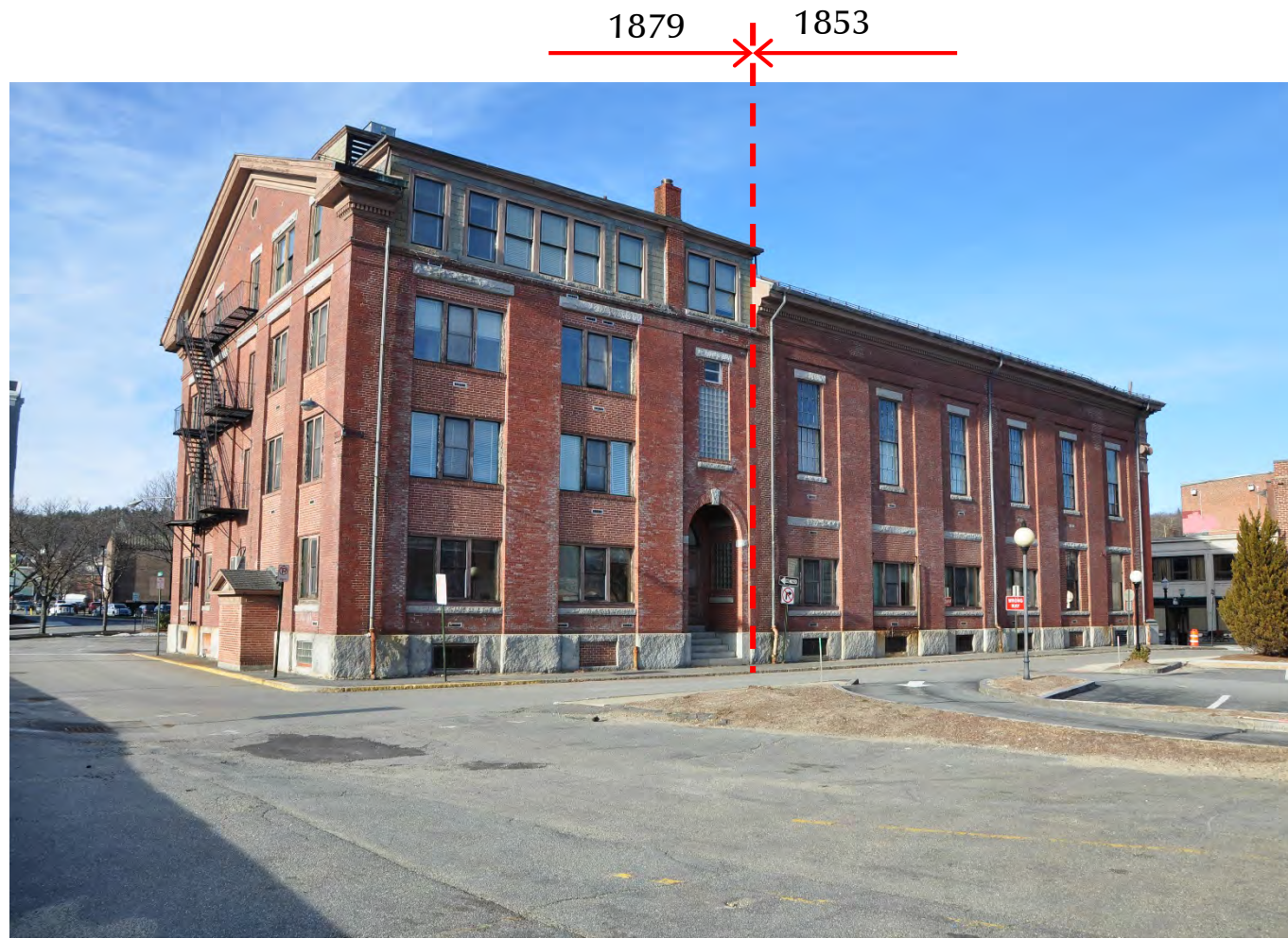
Current View of Building from Southeast
