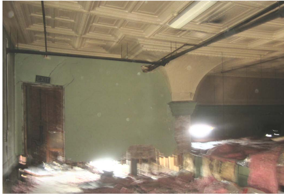
Current View of Existing Attic Space
