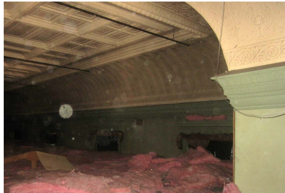
Current View of Existing Attic Space
