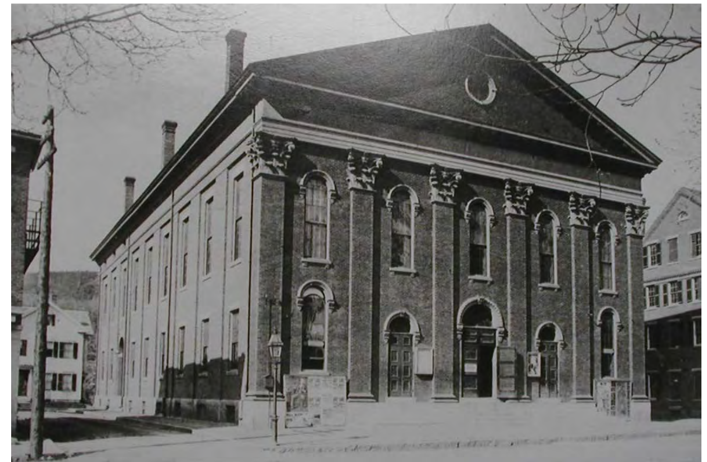
Circa 1879 View of Building from East
