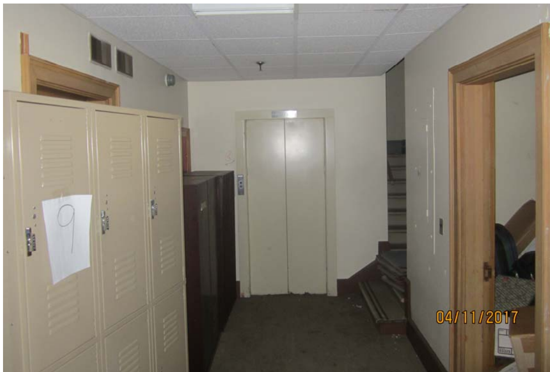
View of interior showing existing elevator and stair
