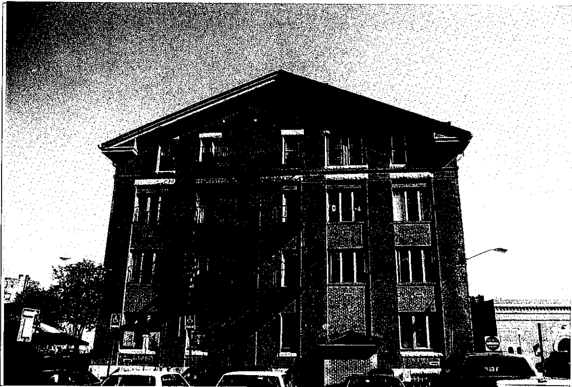
SIDE (REAR) SOUTH ELEVATION
