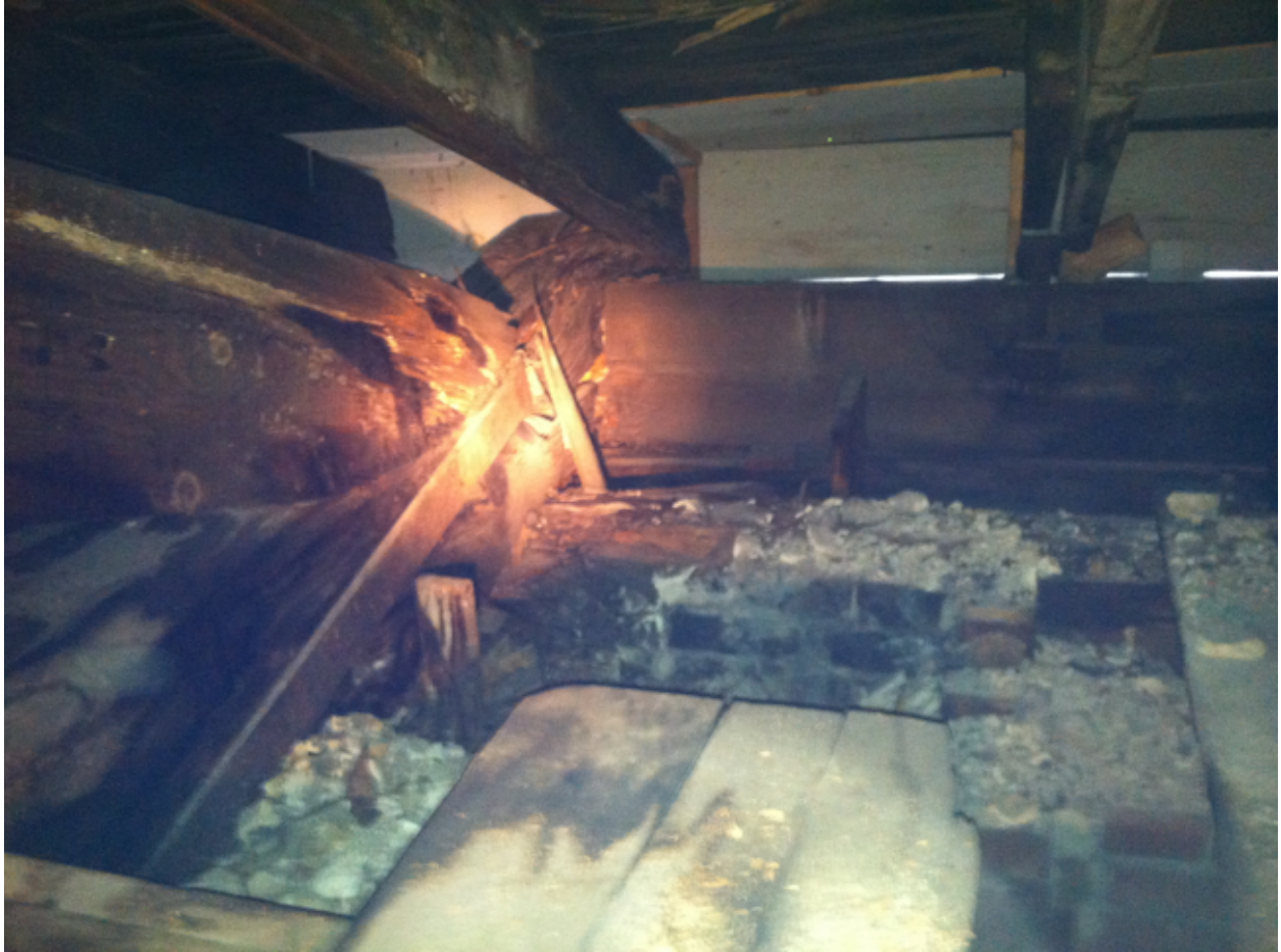
Photograph D: End Bearing of Truss
