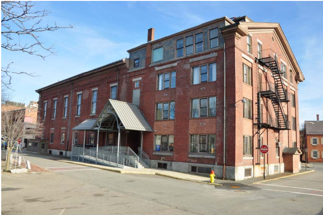
View of exterior from southwest showing existing accessible ramp structure
