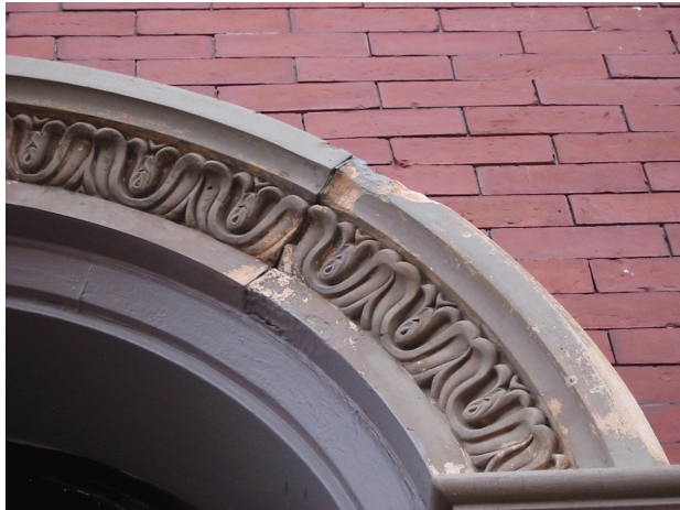
Figure 10: Detailed stone at Main Street entrance.
