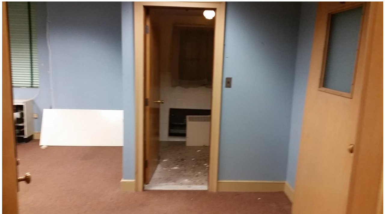
Photo 42 4 th floor – engineering 2 and bathroom
