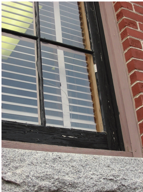
Figure 13: Single pane wood windows.
