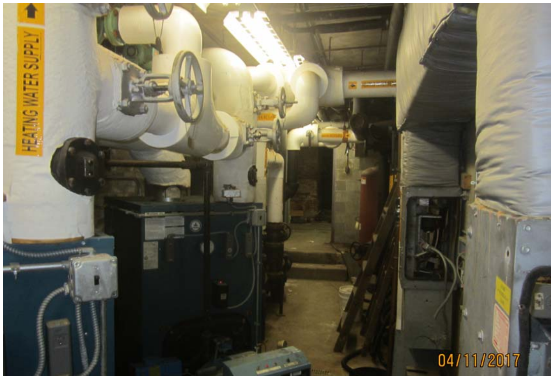
View of existing boiler room
