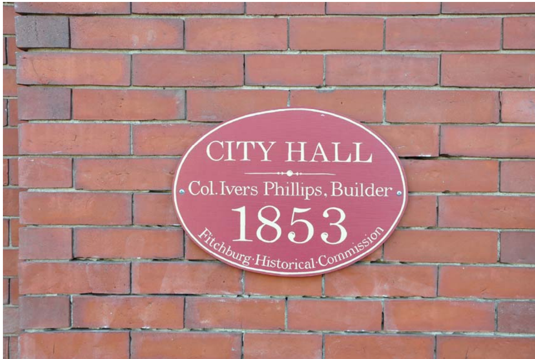
View of typical existing masonry condition requiring repointing
