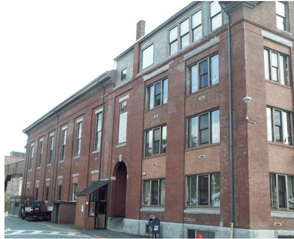
Figure 3: Dormer on west side.
