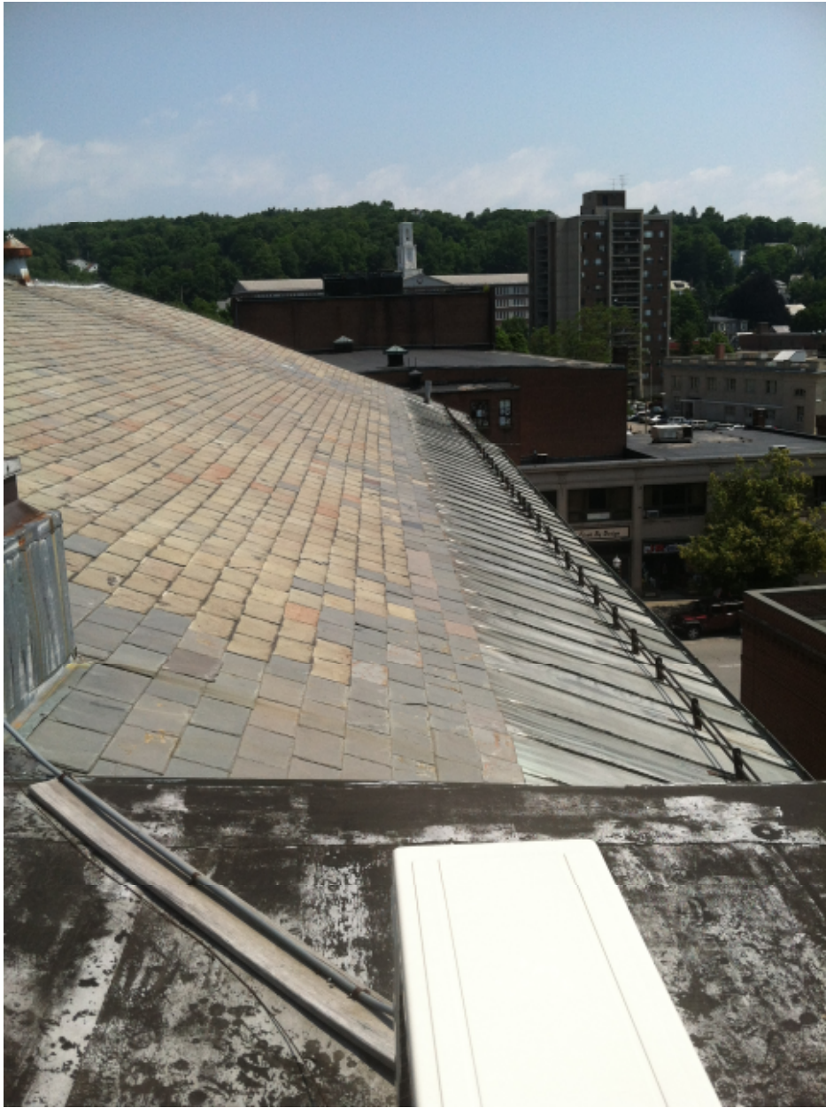
Photograph A: Exterior View of East End of Roof
