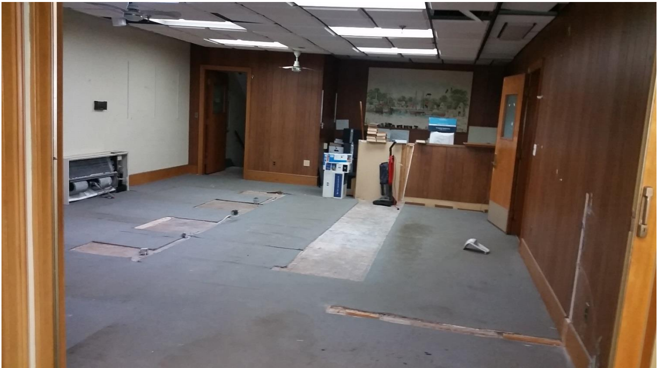
Photo 34 3 rd floor – building 3
