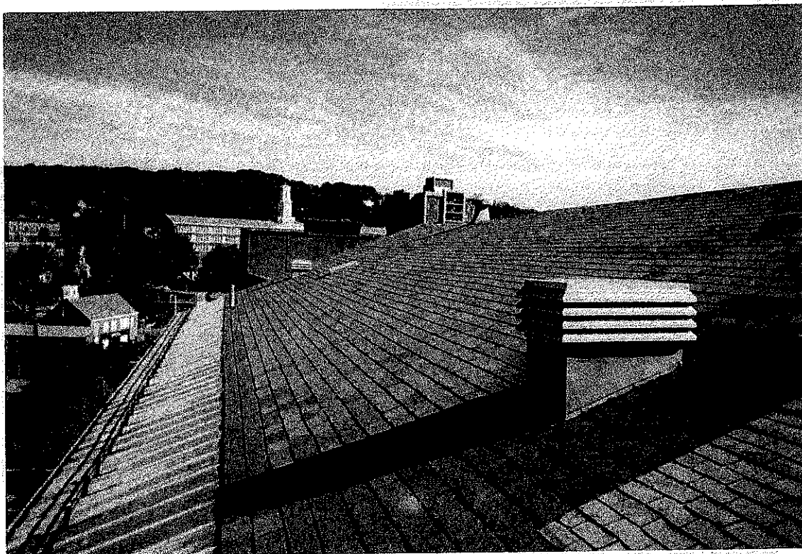
PHOTOGRAPH #4 - WEST SIDE OF ROOF LOOKING NORTH
