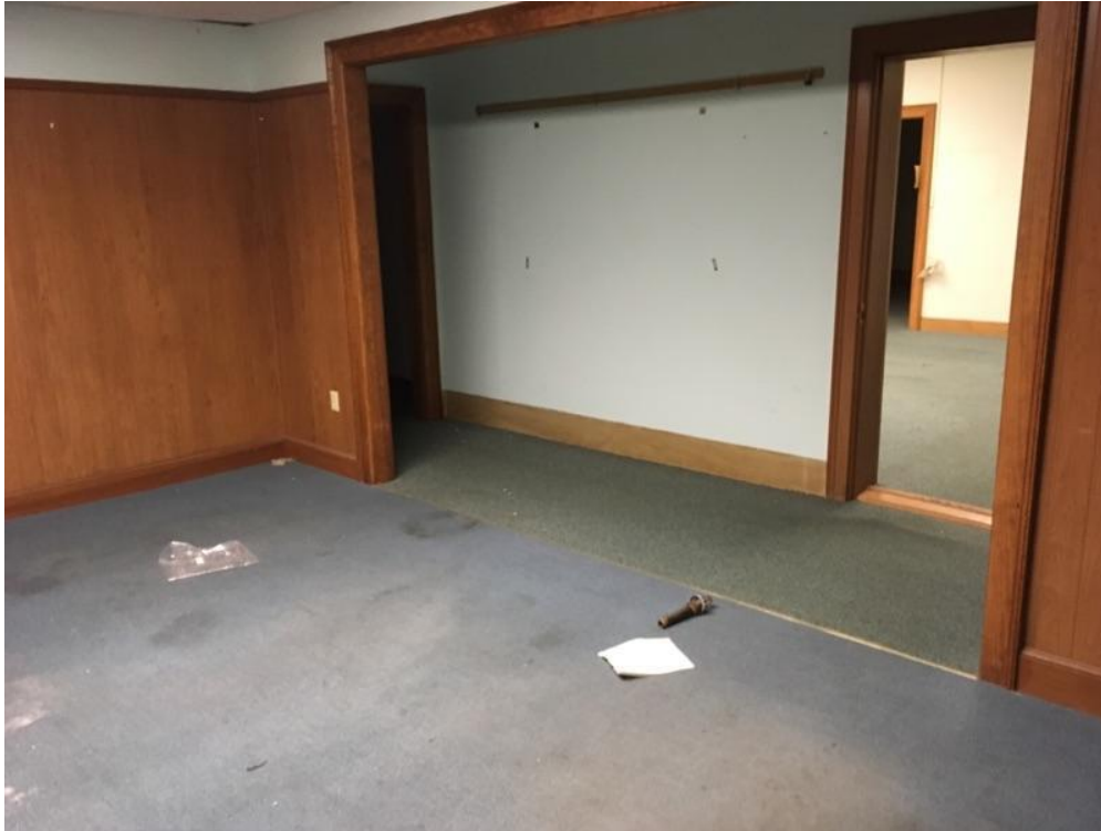
Photo 19 2 nd floor – rear planning
