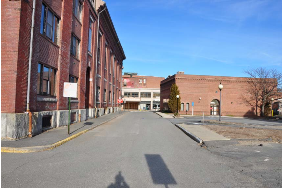
View of exterior looking northeast showing existing paving
