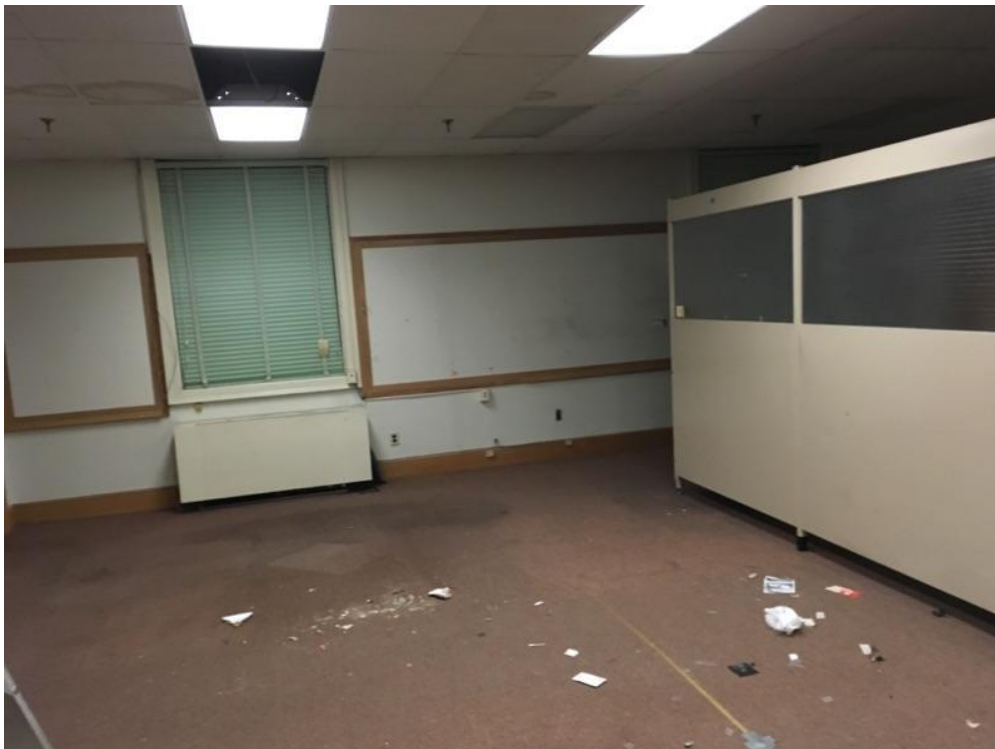
Photo 20 2 nd floor – front planning
