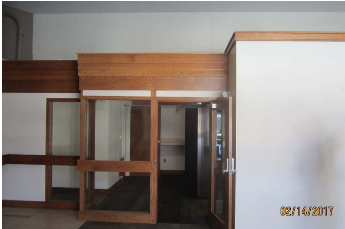
View of bank building interior showing existing vault wall at right
