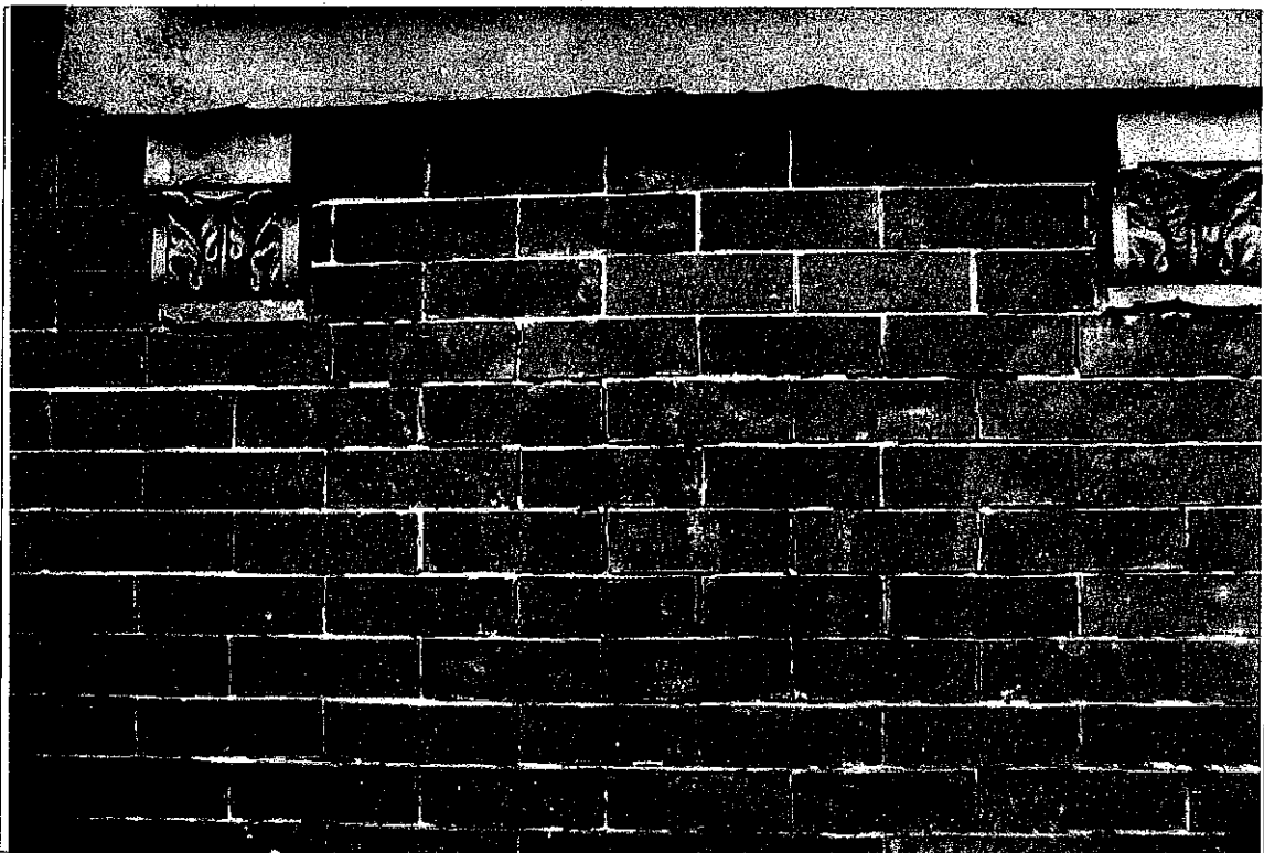
OPEN BRICK JOINTS BELOW SLATE WINDOW STOOL
