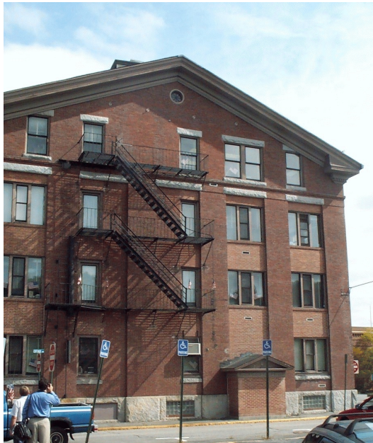
Figure 5: Fire escape on rear wall.
