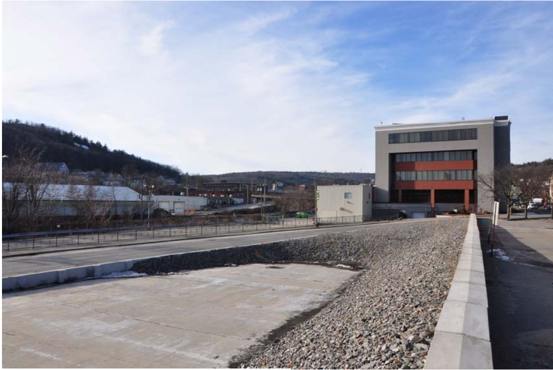
View of demolished parking structure looking west
