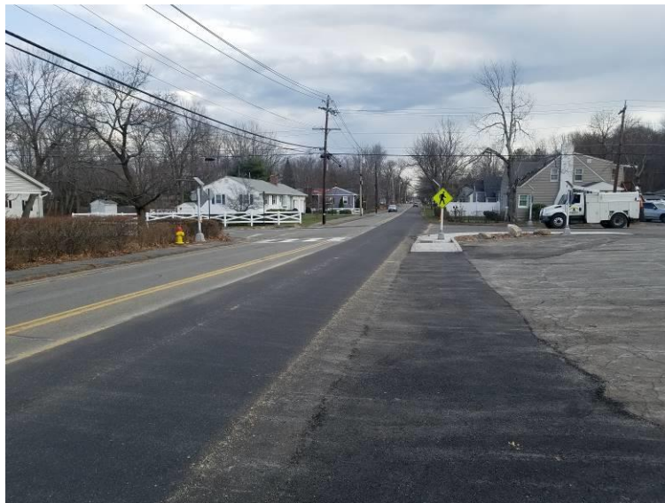
Figure 1 - Paving of UNITIL trenches
