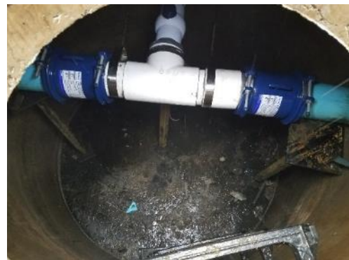
Photo #4: City-performed Force Main Piping Repairs.
