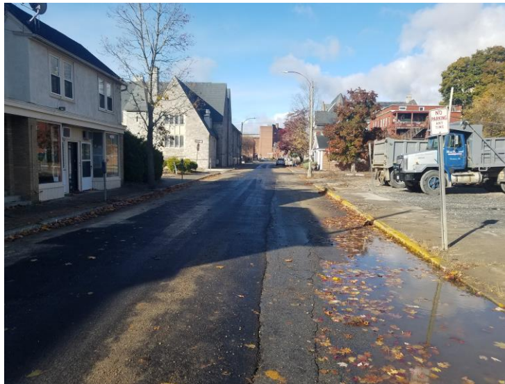
Figure 3 - Elm Street trench paved
