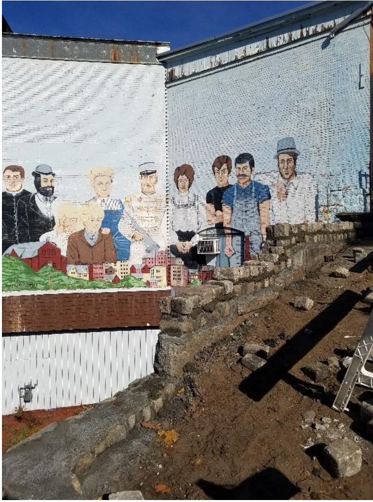
Figure 2 - Sidewalk Crew repairing sidewalk, wall & Fence on Allen Place
