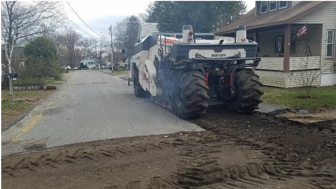
Figure 1 - Pulverization of Garfield St
