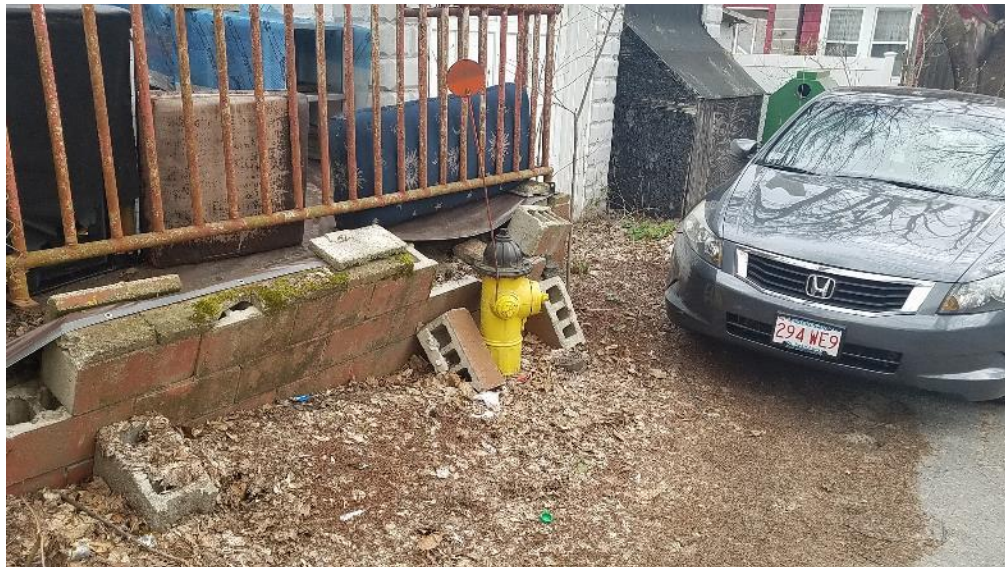
Figure 3 - Hydrant blockage
