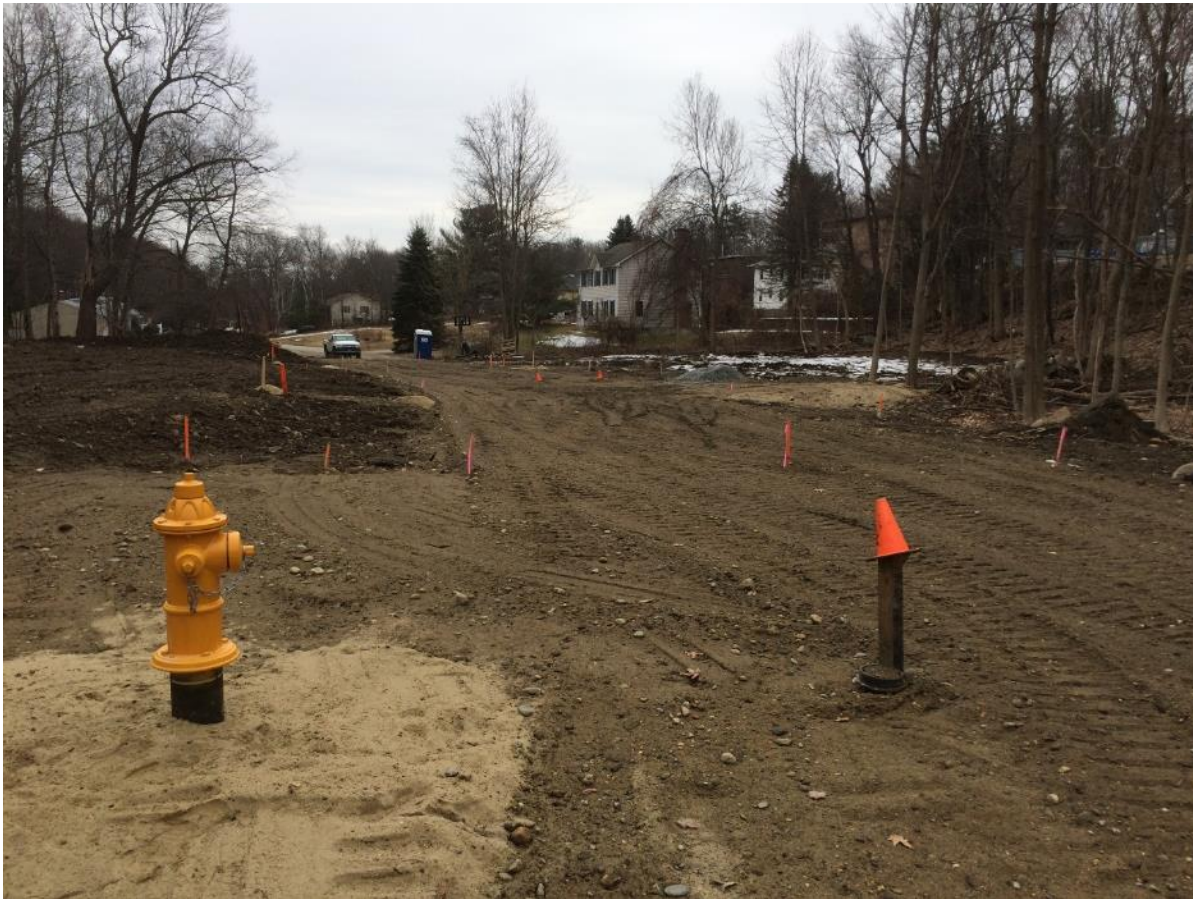
Figure 1 - Valley St. Extension project
