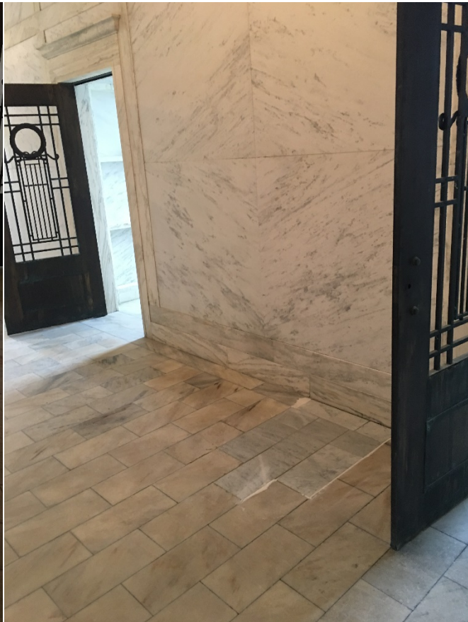
Mausoleum Floor Repairs
