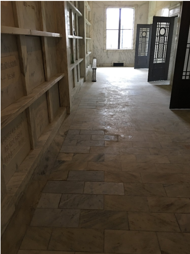
Mausoleum Floor Repairs
